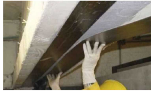
Figure 6.3.3 Example of Continuous Fiber Plate Bonding Method
