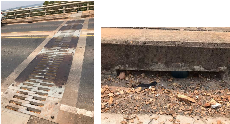
Figure 3.2.1 (Left) Expansion Joint, (Right) Drainage
