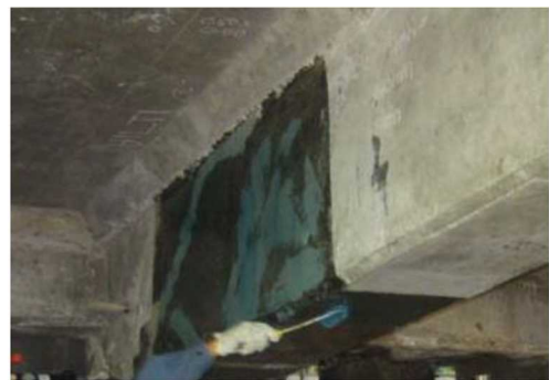
Figure 6.3.2 Example of Shear Strength Reinforcement
