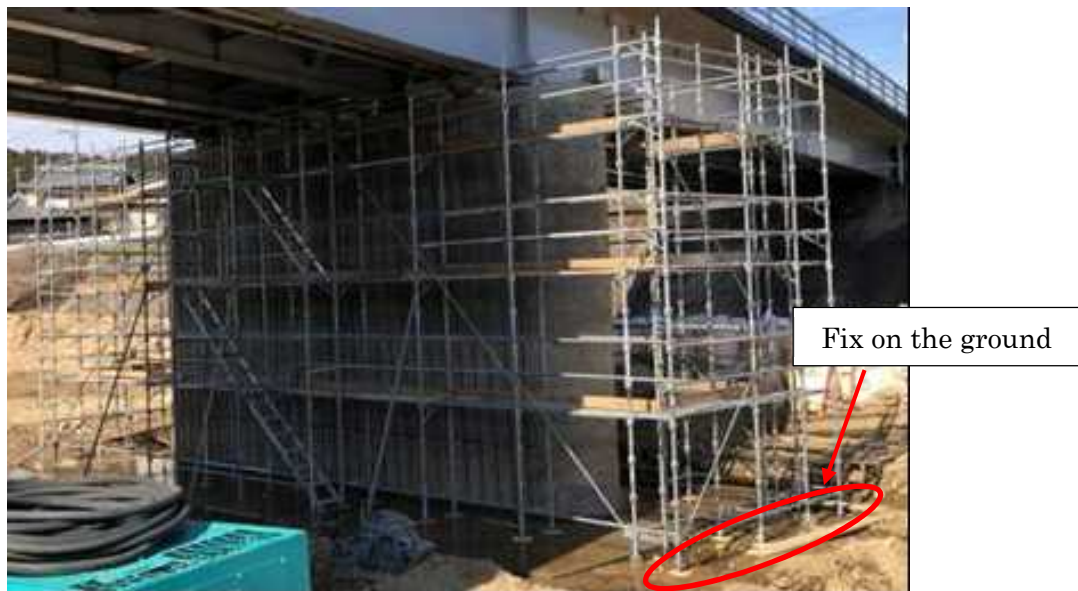
Figure 3.1.7 Fixed Scaffolding
